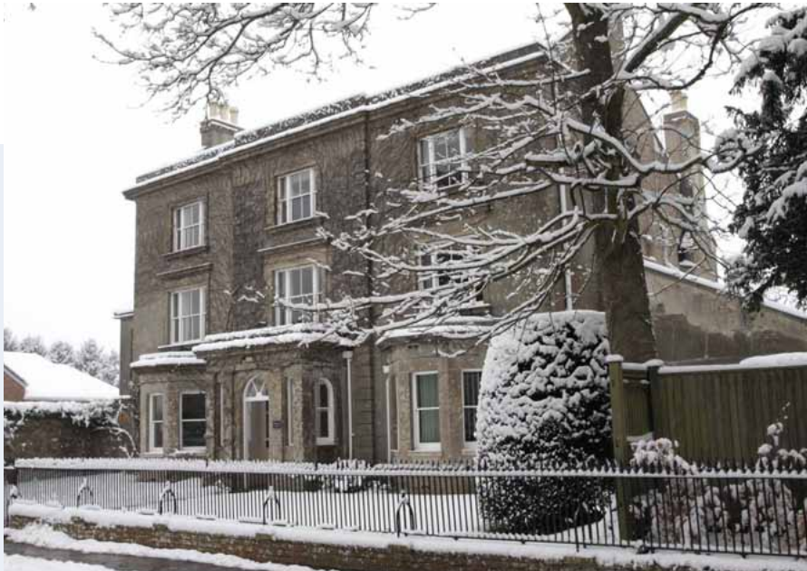
SOUTHWICK ESTATE OFFICE
